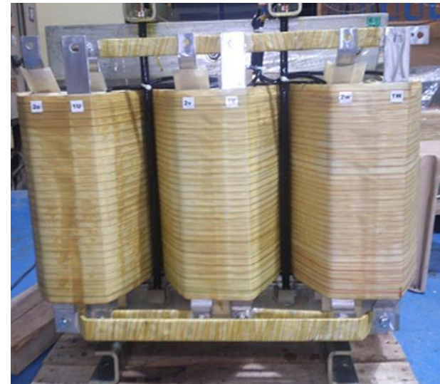
150 KVA Transformer (UPS)
